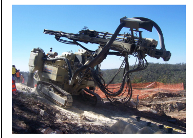
Photo: Trackdrill working at the spillway site, Shannon Ck Storage 11/7/07
